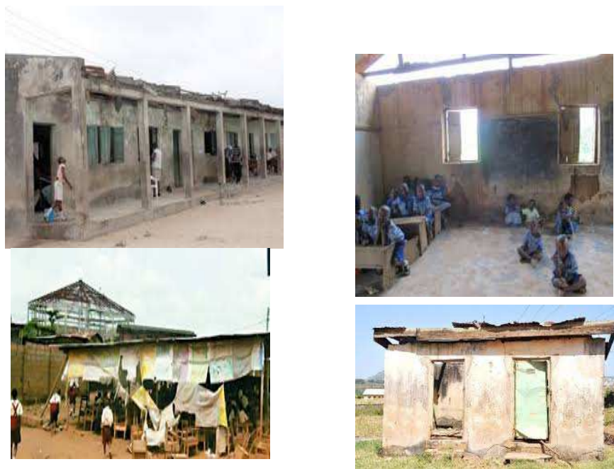
Figure 2: Typical Nigerian School Environment
